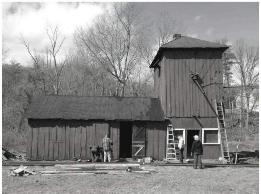
“This bin forms the upper section of the sand house, the ‘tower.’ It is made with a sloped bottom, to feed into the lower loading pipe or out the drain. The bin had two outlet pipes, one up high for filling a locomotive's sand dome, and another, lower pipe for loading sand into boxcars. These would be hauled to Saltillo or Robertsedale for use in refilling the locomotives there. Both of these loading pipes had air jets to help move the sand.”
